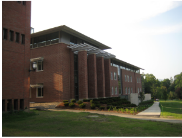
North Academic Building – View of Aluminum Trellis and Aluminum Sunshades
